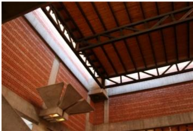
Figure 9. Roelof Uytenbogaardt. DRC Welkom West. 1964. View of ceiling 2009. (photo by author)
